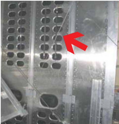
Swing-to-roof elevation cable in use.
