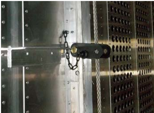
Raise Empty Deck Above Supports and Lower Support with Pin
