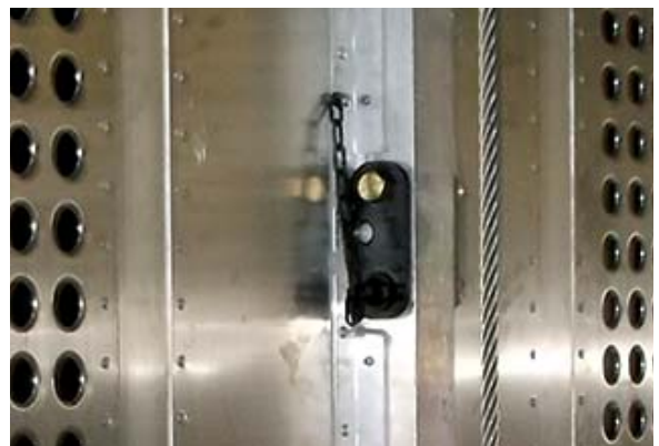
Manual Deck Support Stored
