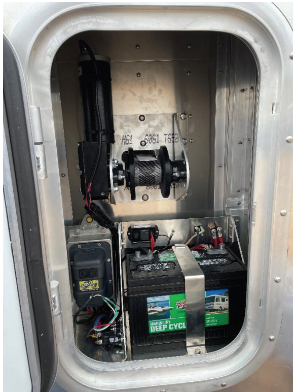
Electric hoist, controller, and battery (located on the front of trailer)
